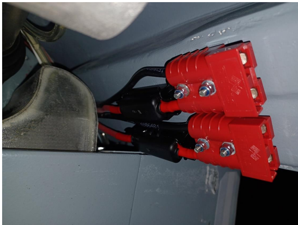
Fig. 3 – Replacement cable after installation.
